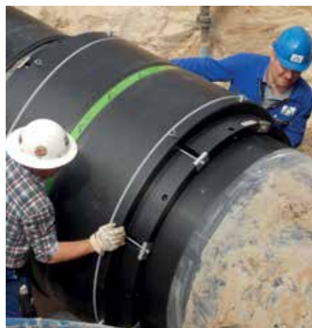
Conical ring coupler KM XL can be pushed on with ease.
