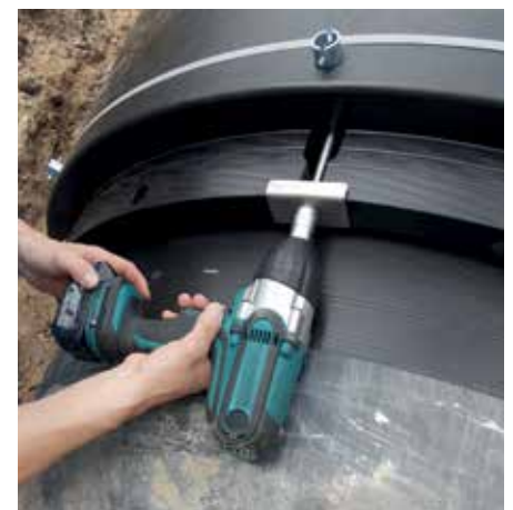
Conical ring activated with a cordless screwdriver
