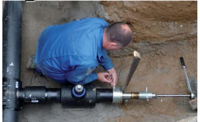
Picture 3: Drilling via standard flange, valve and SAFL
