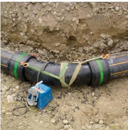
■ The PE elbows were fused using a FRIAMAT fusion unit
