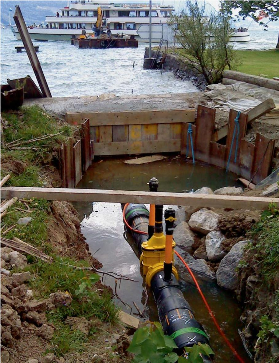
■ Connection of a shut-off valve at the transition land / sea
