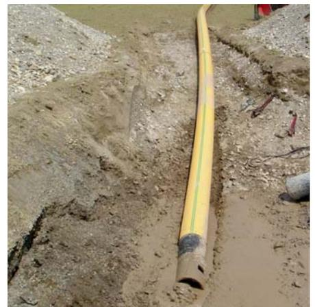
■ Preparation of the insertion of a pipe section into the horizontal flush drilling
