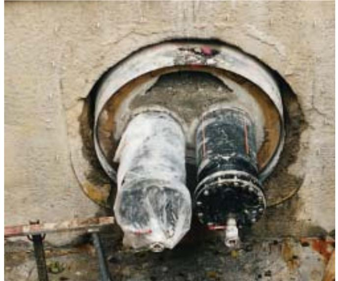
Picture 5: HDPE pipe run surrounded by light pore concrete
