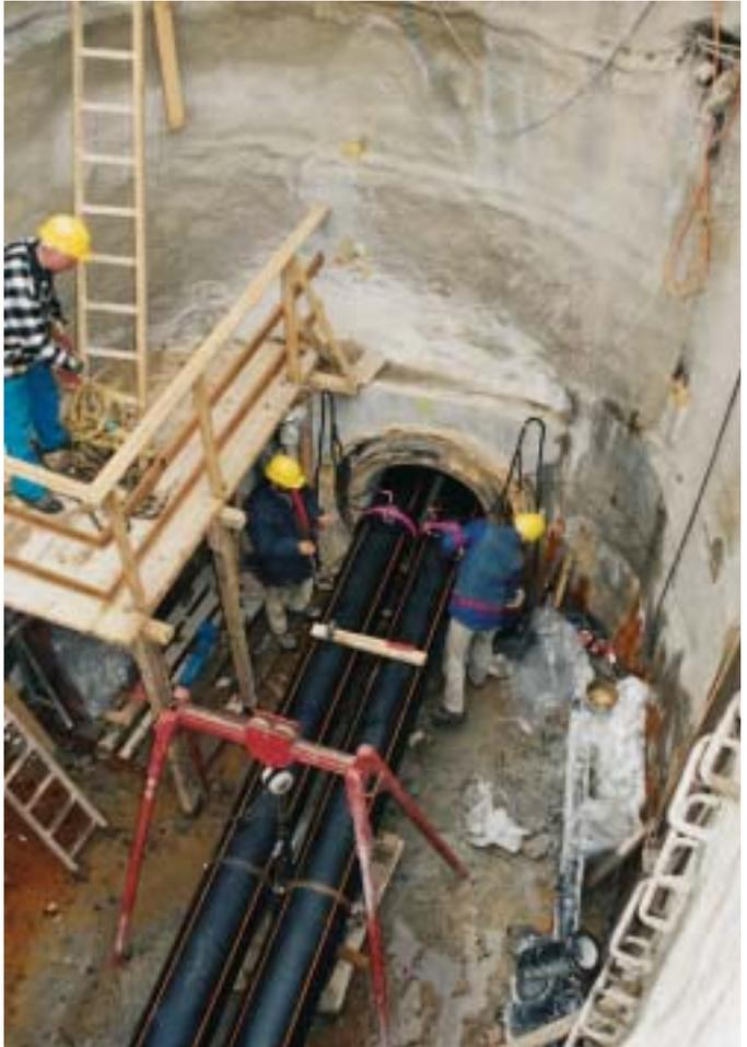
Picture 1: HDPE pipes, 6 m long, in twin pack, in 8 m deep hole
