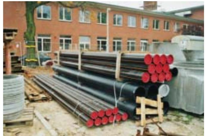
Picture 2: HDPE pipes and inspection chambers just before installation
