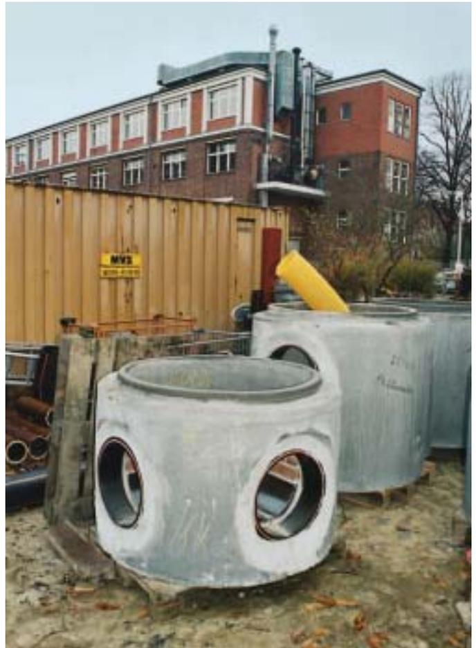
Picture 4: Inspection chambers furnished with FRIAFIT® inspection chamber adapter
