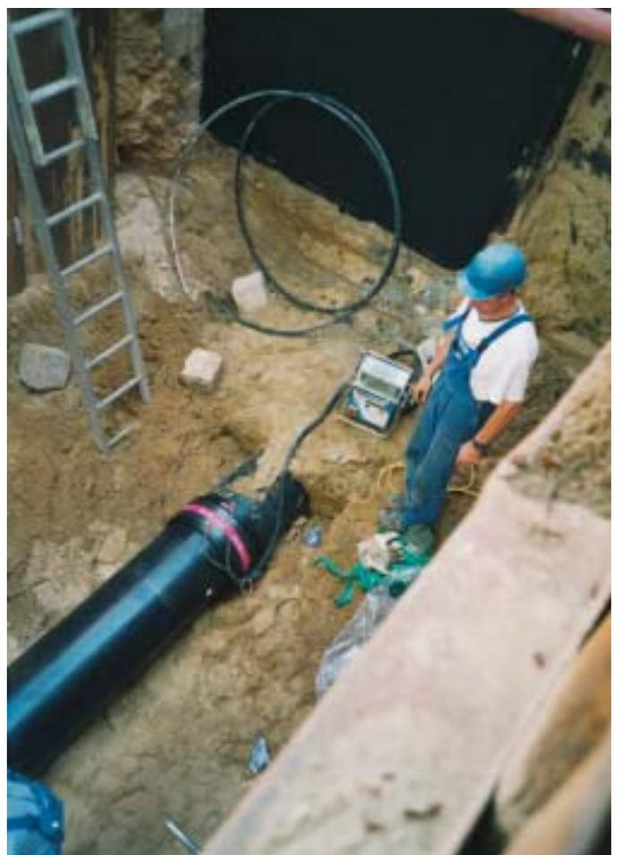
Picture 5: Fusing a FRIAFIT® coupler d 450
