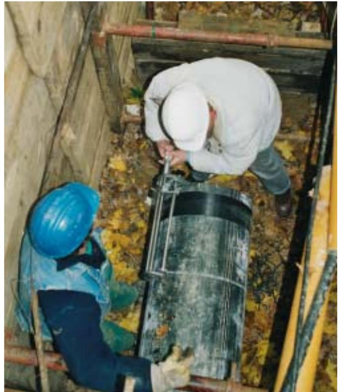
Picture 6: Demonstration on site: scraping of a HDPE pipe d 450 using FRIATEC scraper tool FWSG 630
