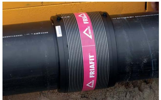
Fig 2b - Completed pipe connection
