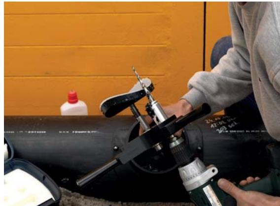
Fig 3b - Pipe cutout being removed
