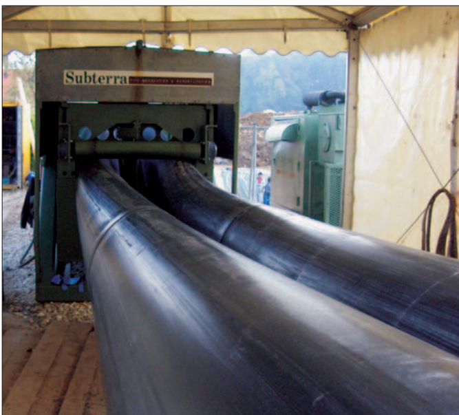
Fig. 5: Folding of the PE-liner
