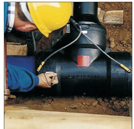
Fig. 2: Resistance welded fittings in the form of a T-junction or elbow up to d 225 provide potentials for cost-savings
